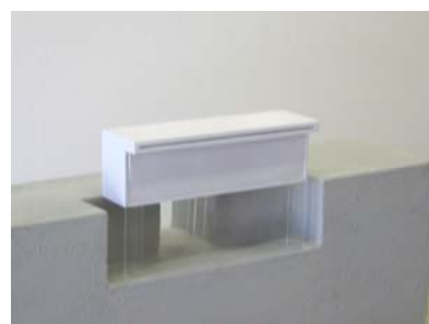
Set the unit into the front side of the wall.
